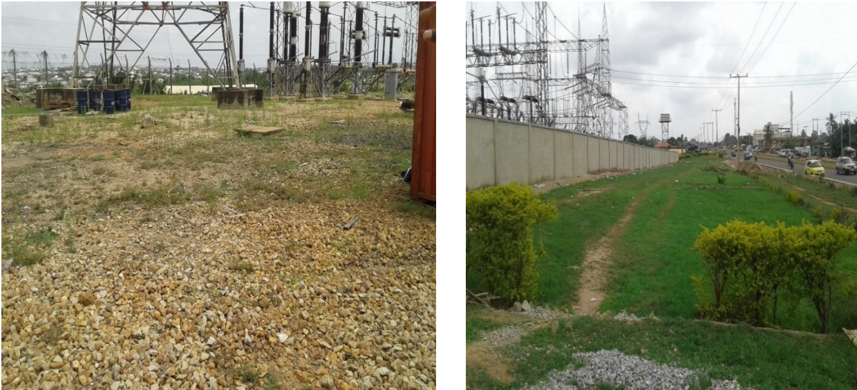
Figure 9: Weed overgrowths within the switchyard/Weed overgrowths within the switchyard.
