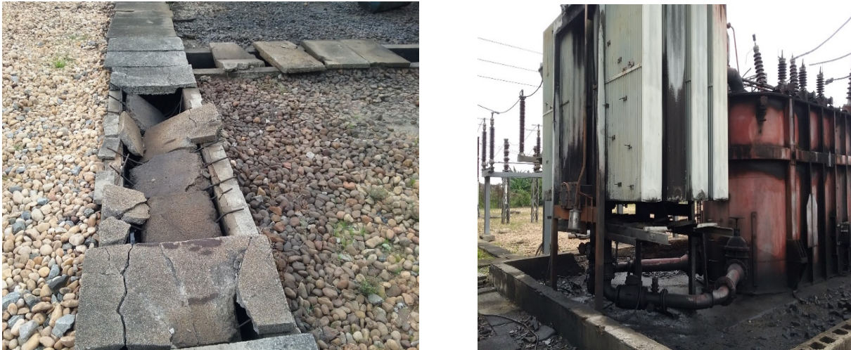
Figure 40: Broken/Collapsed trench slabs and Spilled oil from very old transformer within switchyard.
