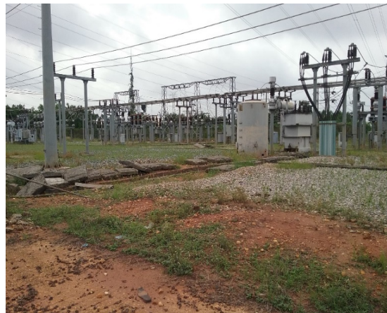
Figure 23: Overgrown weeds have taken over part of the Switchyard floor/Part of Switchyard floor with scanty gravelling.
