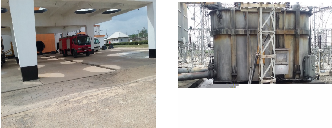
Figure 20: Standard standby fire-fighting truck within the substation premise. /Spilled oil from an old .
