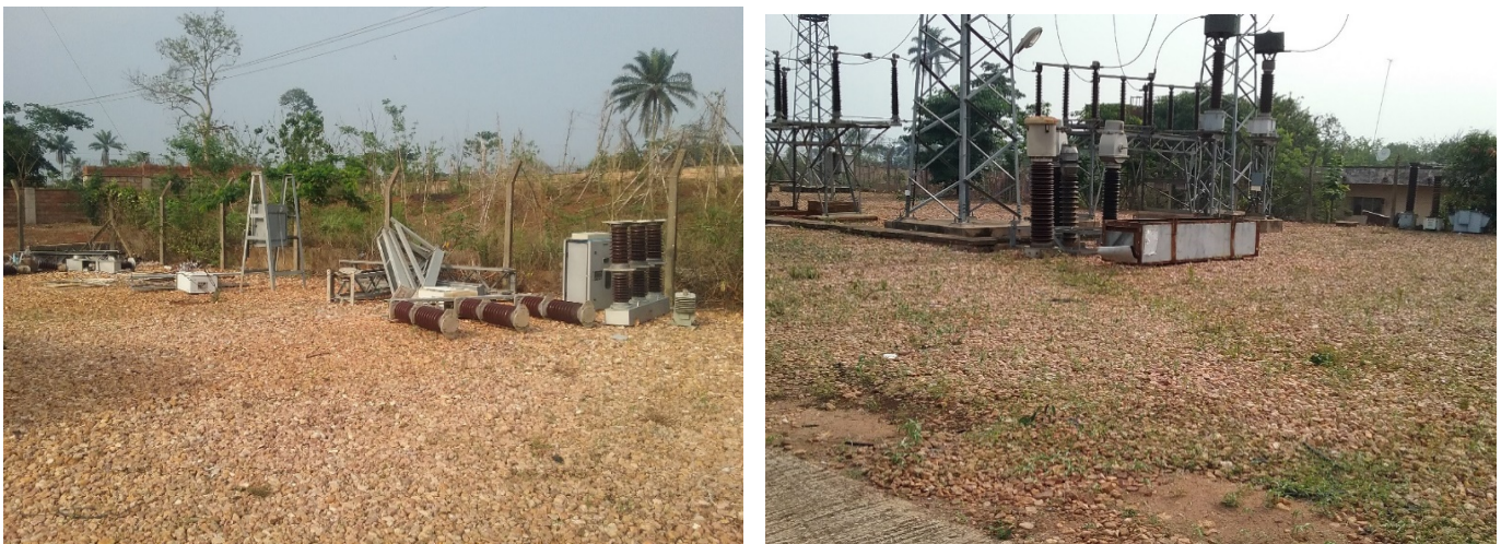
Figure 35: Scraps littering the Substation premise/ scantily graveled switchyard floor (with patches of light overgrowths).
