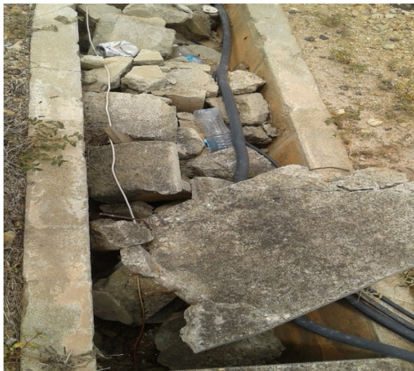
Figure 12:Blocked drainage channels/Transformer base showing signs of slight oil leakage.
