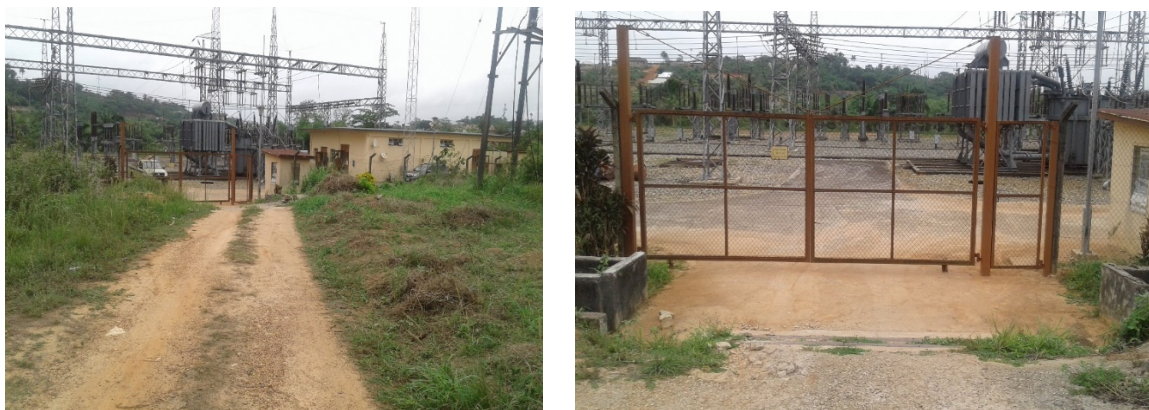
Figure 31: Approach to the substation entrance/Rusty and weak looking entrance gate Securing the substation.
