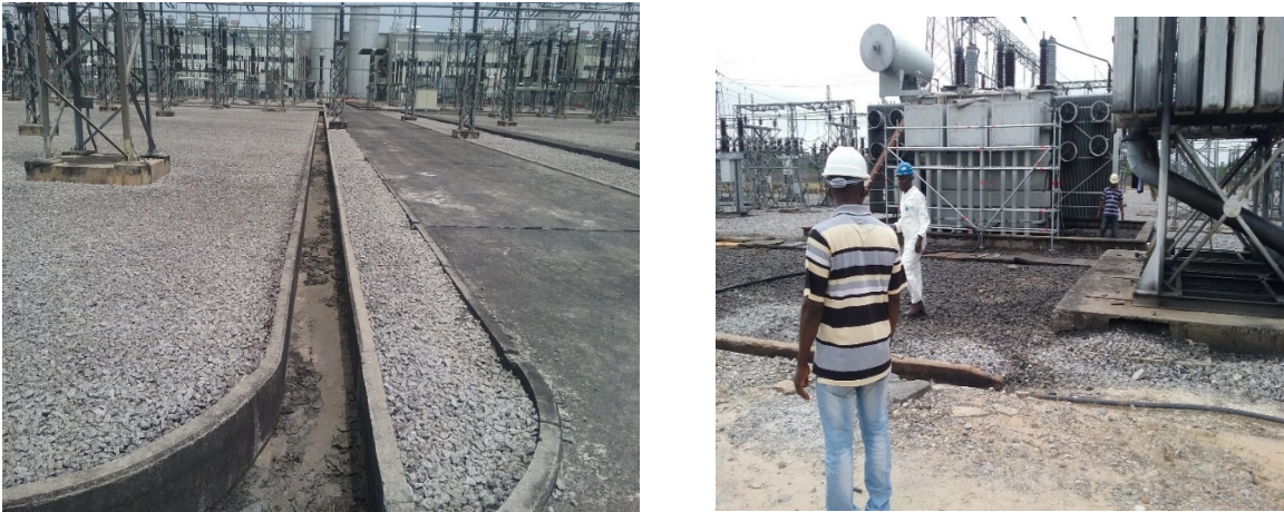
Figure 19: Well-maintained drainage channel/Strict adherence to use of PPEs during operations. .
