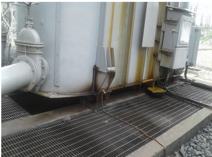
Figure 32: Transformer base showing signs of oil leakage.
