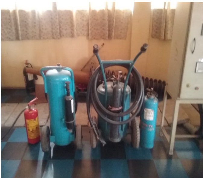
Figure 41: Fire Extinguishers at the Control Room.
