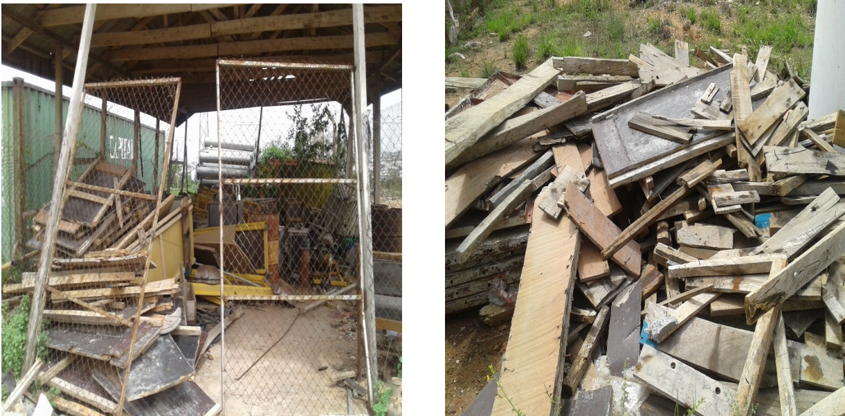
Figure 10: Temporary designated Junkyard / Scrap generated from on-going construction works.
