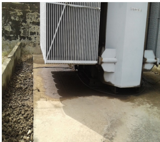
Figure 28: Antiquated generator in use at the Substation (source of noise and air pollution)/Transformer base showing signs of oil leakages.
