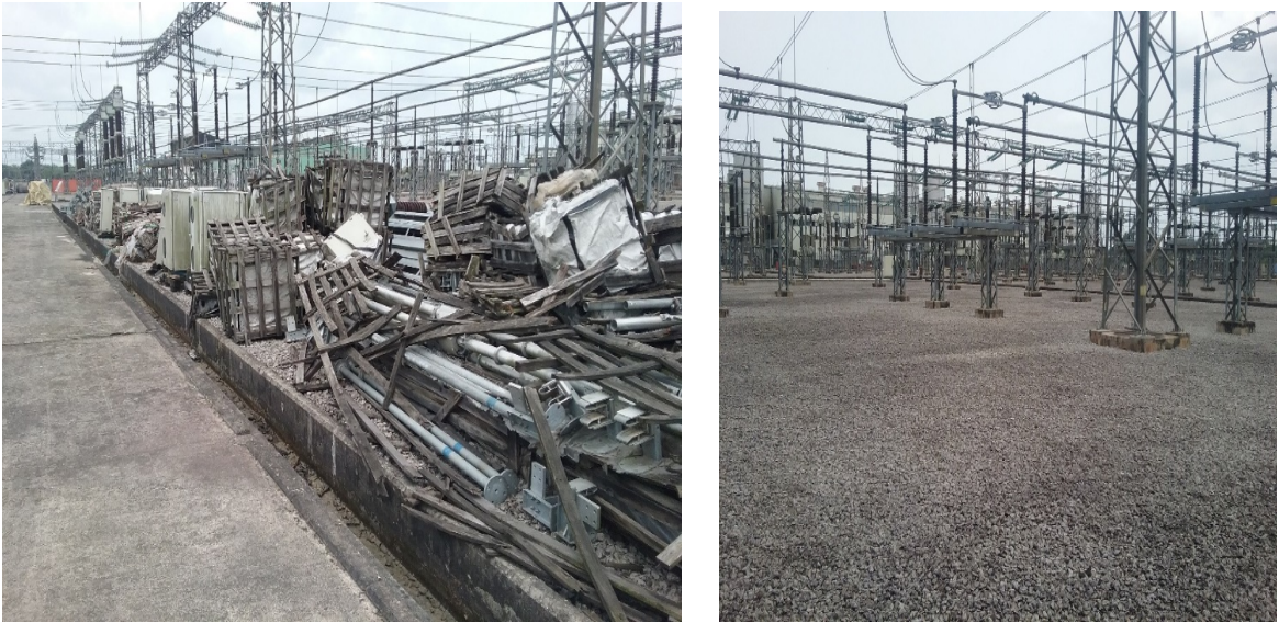
Figure 18: Abandoned unused installation materials/Properly maintained Switchyard floor.
