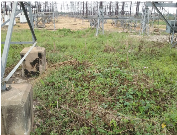
Figure 23: Overgrown weeds have taken over part of the Switchyard floor/Part of Switchyard floor with scanty gravelling.
