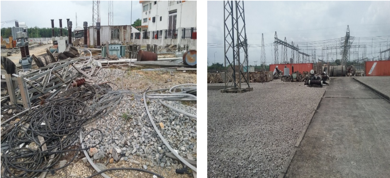
Figure 17: Improperly disposed waste materials/Decommissioned equipment/materials littering the Substation premise.
