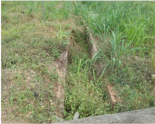
Figure 24: Blocked drainage channel completely overtaken by overgrowths/Strict adherence to use of PPEs during application of weed control chemical fumigation.
