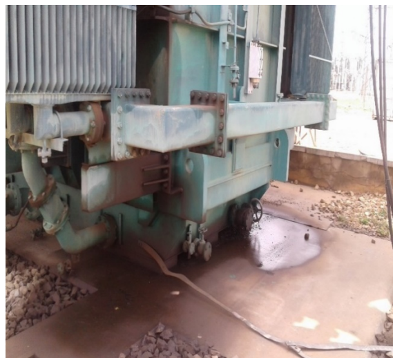
Figure 12:Blocked drainage channels/Transformer base showing signs of slight oil leakage.
