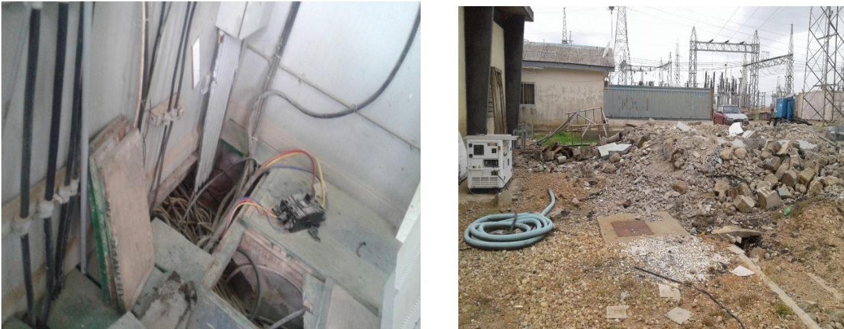
Figure 13: Exposed cable trenches within the Control room/Debris of demolished building
