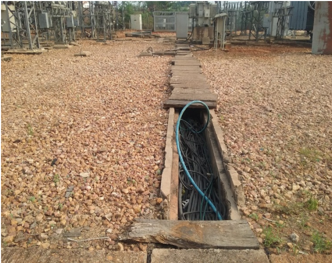
Figure 36: Missing cable trench slabs.
