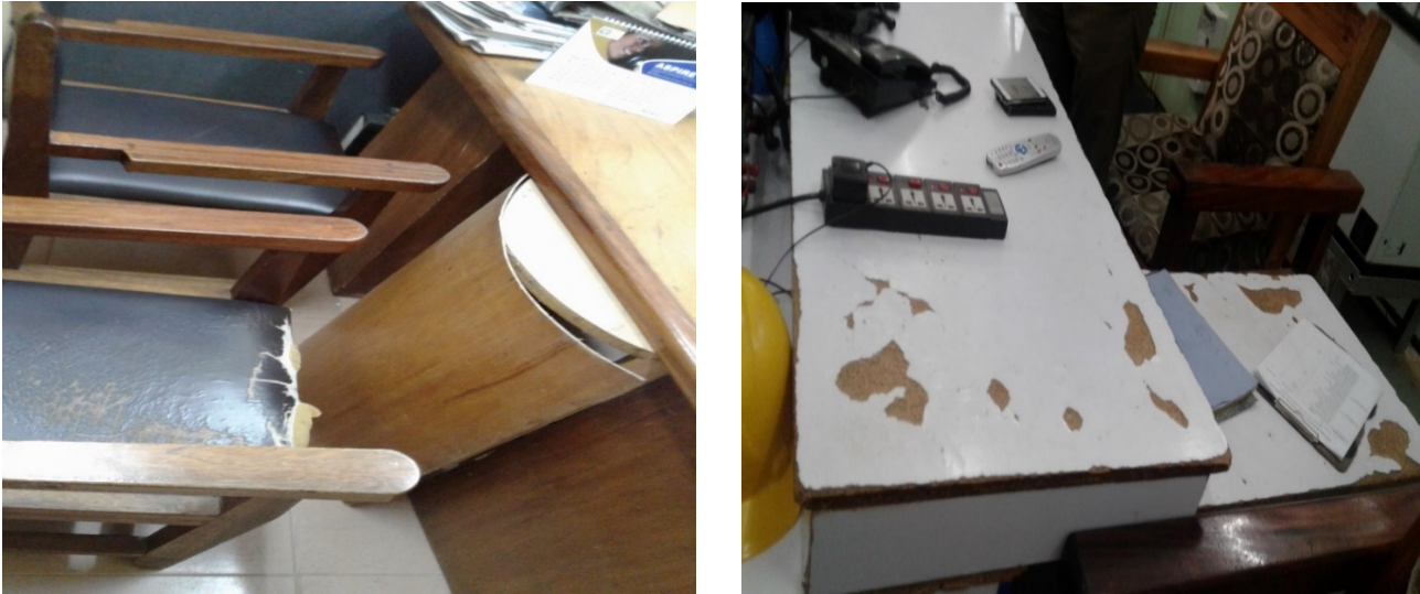
Figure 14: Bad office furniture available for use by operators /Decaying work table in use by Operators
