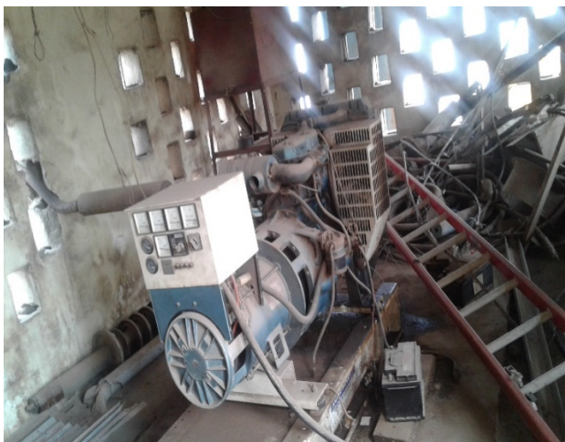
Figure 28: Antiquated generator in use at the Substation (source of noise and air pollution)/Transformer base showing signs of oil leakages.
