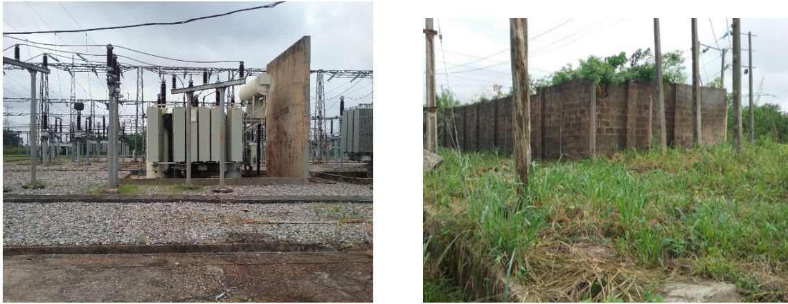
Figure 26: Oil Spill-free transformer base/Fenced-in Shrine within the substation premise
