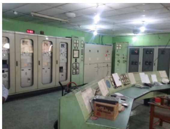
Figure 16: Substation Control Room is domiciled/Control panels in the existing Control within Transcorp Power building.
