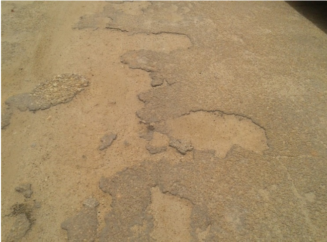
Figure 11: Drive-way within the substation in a bad state.
